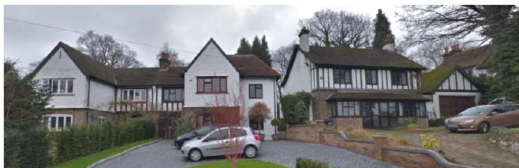
57 & 59 Higher Drive with brick plinths, rendered upper storeys, plain clay roof tiles and casement windows. Both display half timbering typical of imitation Arts & Crafts.
