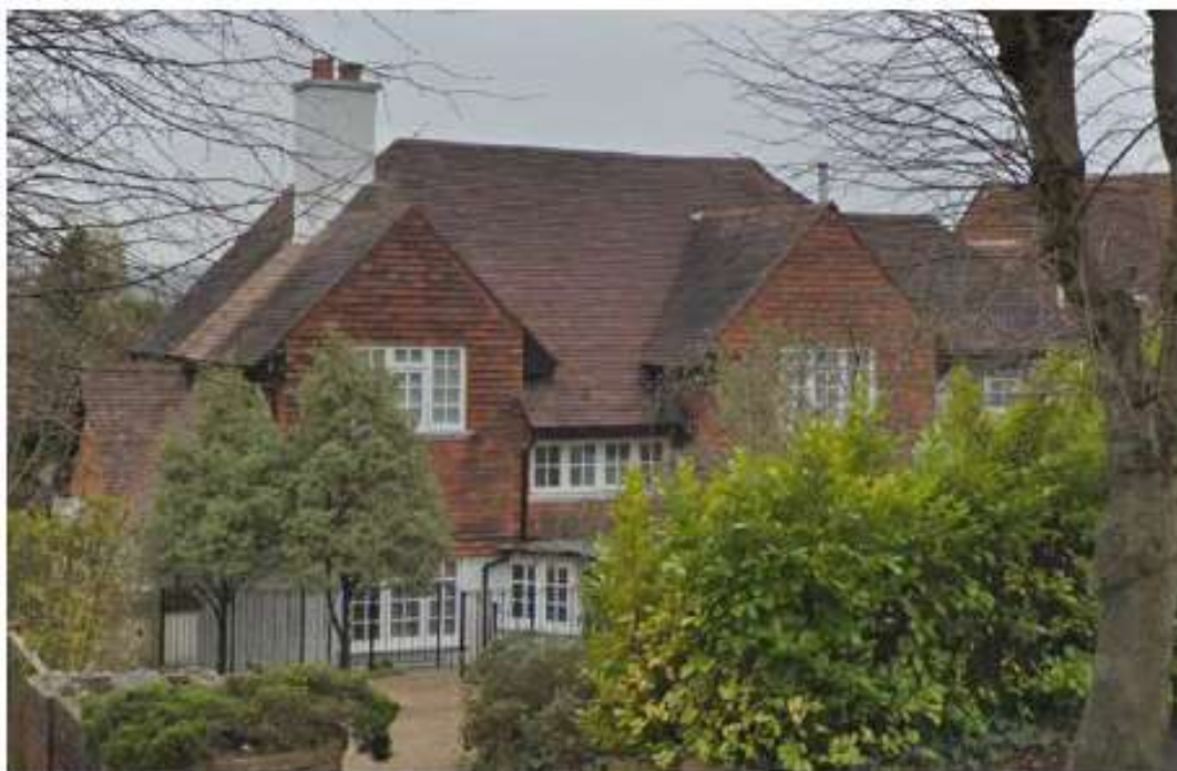
74 Higher Drive with plain clay roof tiles & overhanging eaves, hung tile & render wall treatments and casement windows.
